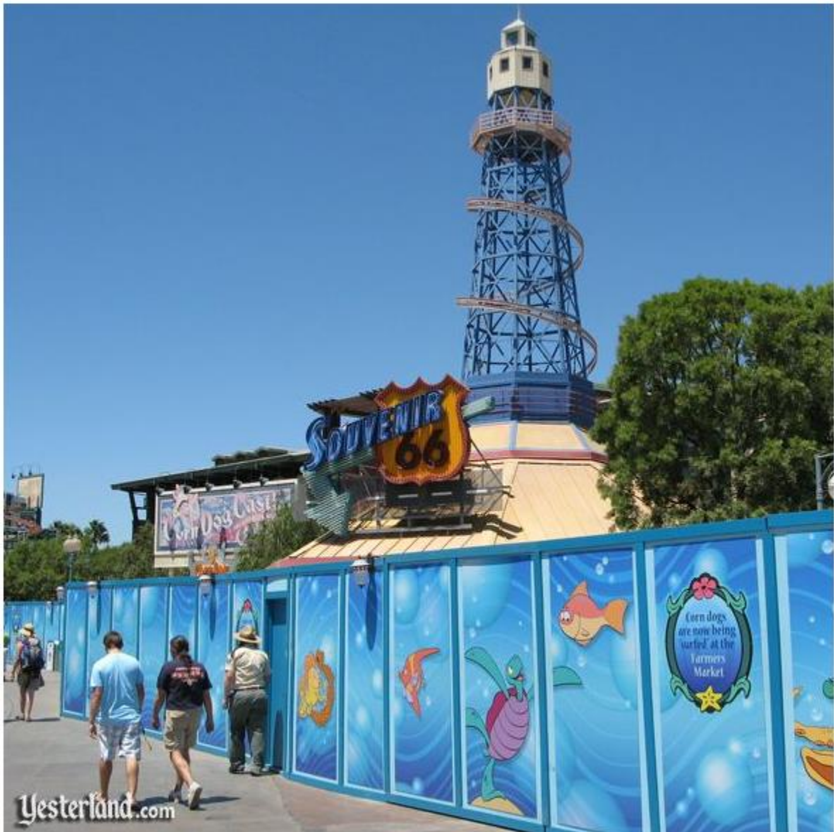
Corn Dog Castle and Souvenir 66 behind a construction wall on August 6, 2009
