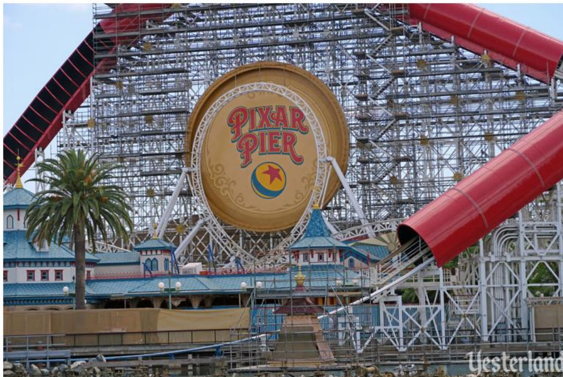
Pixar Pier transformation underway
