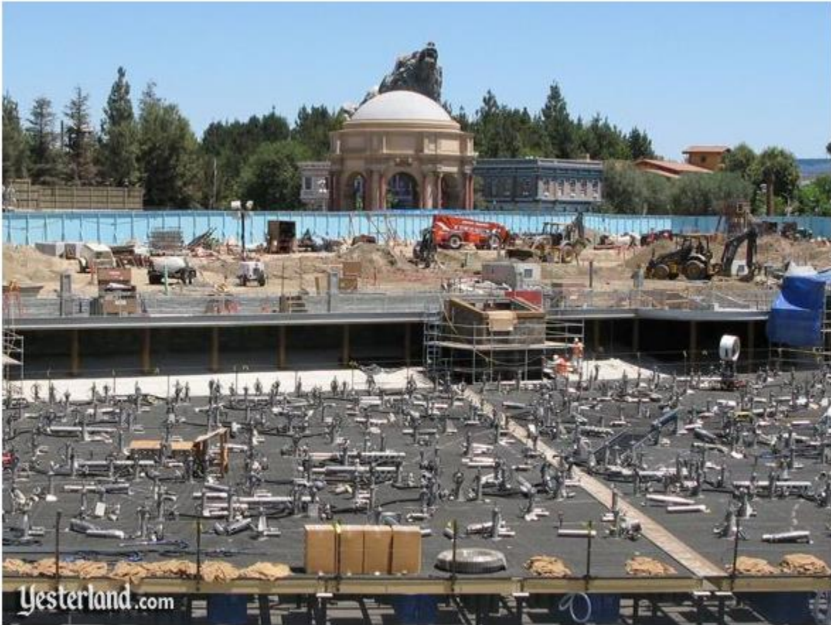
Construction for Walt Disney's World of Color in August 2009
