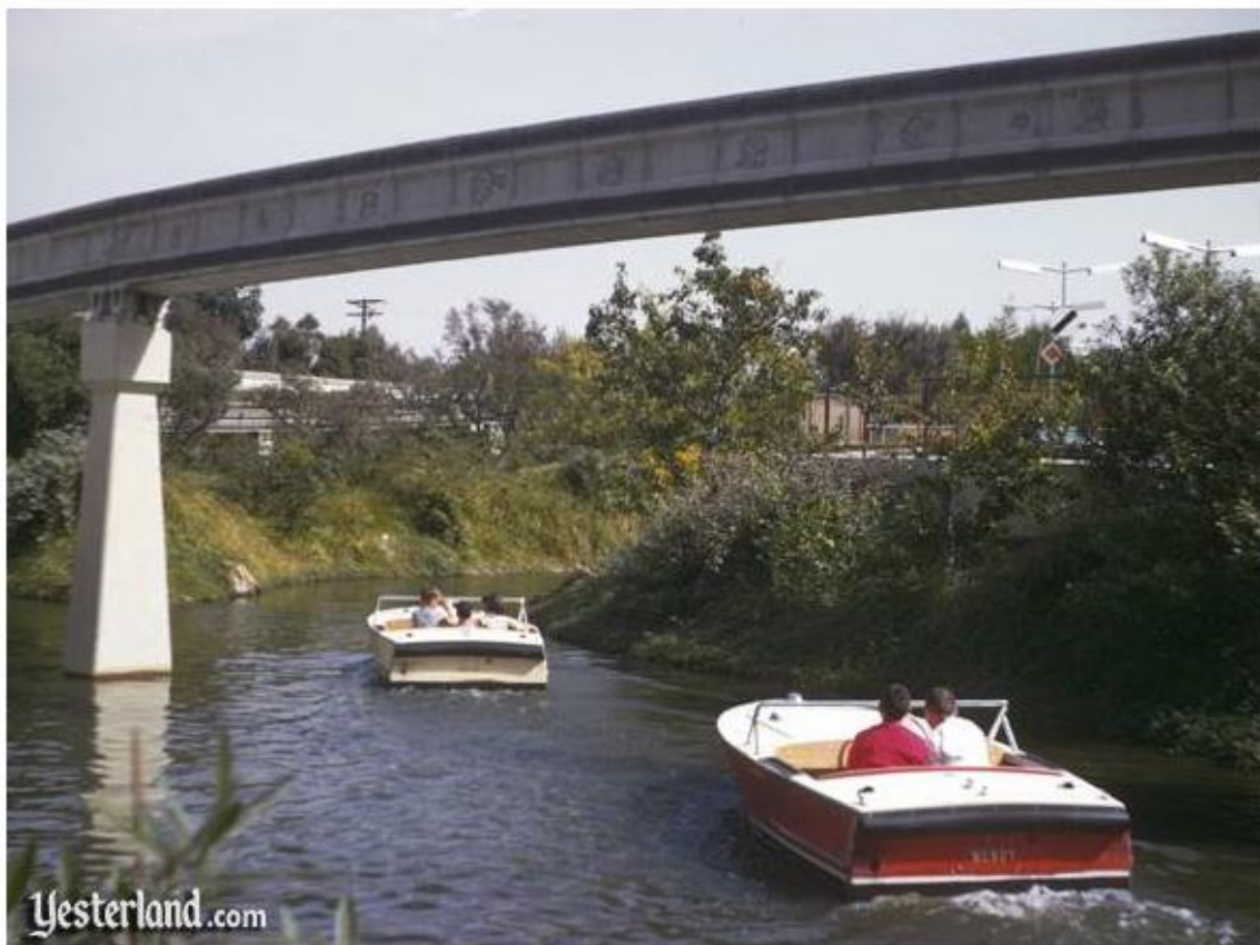
The Disneyland Alweg Monorail beams were added in 1959.
