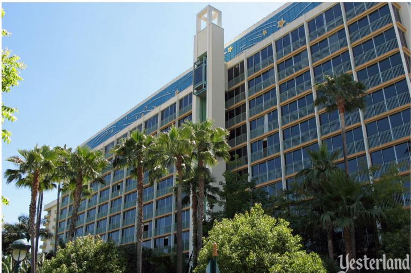
Faux balconies with sliding glass doors, allowing each room to function as a balcony
