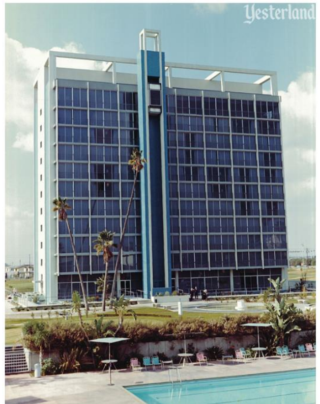
Elevator cab at the top
